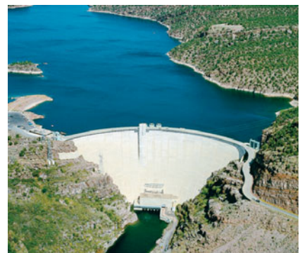
FIGURE 15–27 Problem 55: Flaming Gorge Dam on the Green River in Utah.
