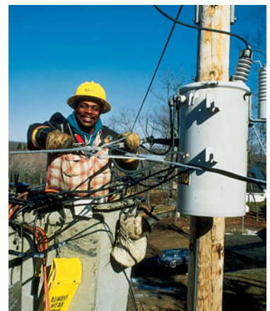
FIGURE 21–22 Repairing a step-down transformer on a utility pole.
